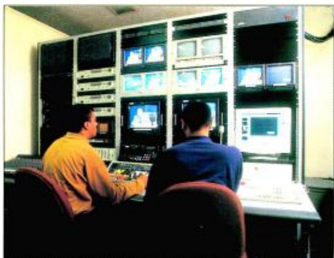
One of the two NOAT control rooms. Louth Automation and the Grass Valley model 101 master control switcher are shown.
